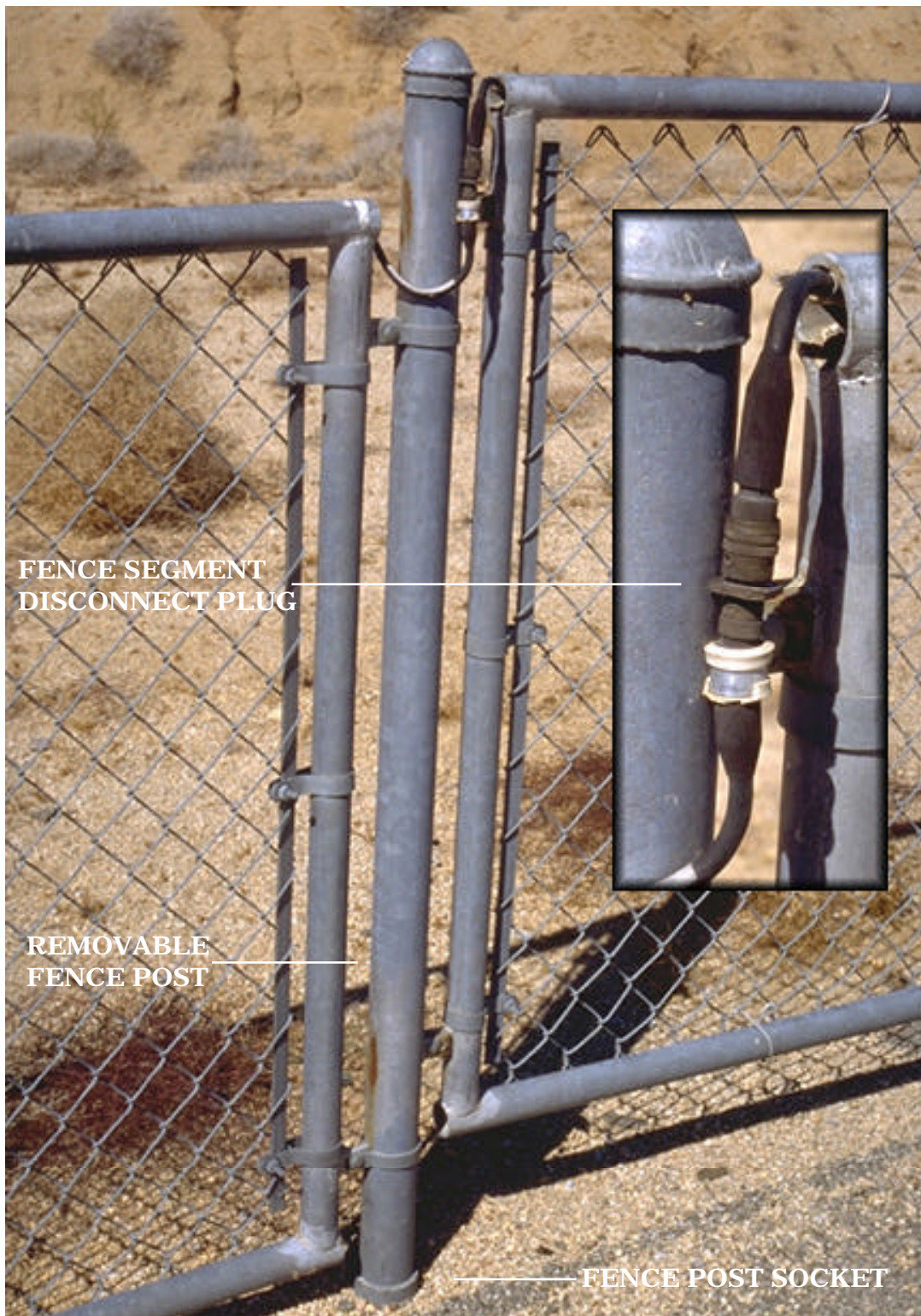
GAVRT ANTENNA PERIMETER INTEGRITY FENCE
