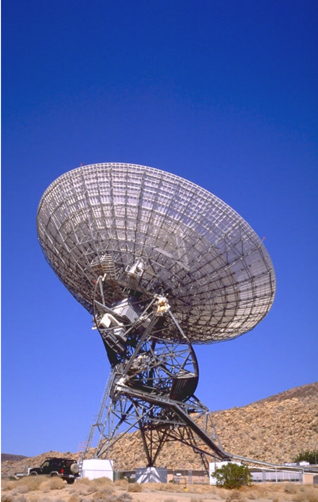
GAVRT ANTENNA AT NORTH LIMIT
